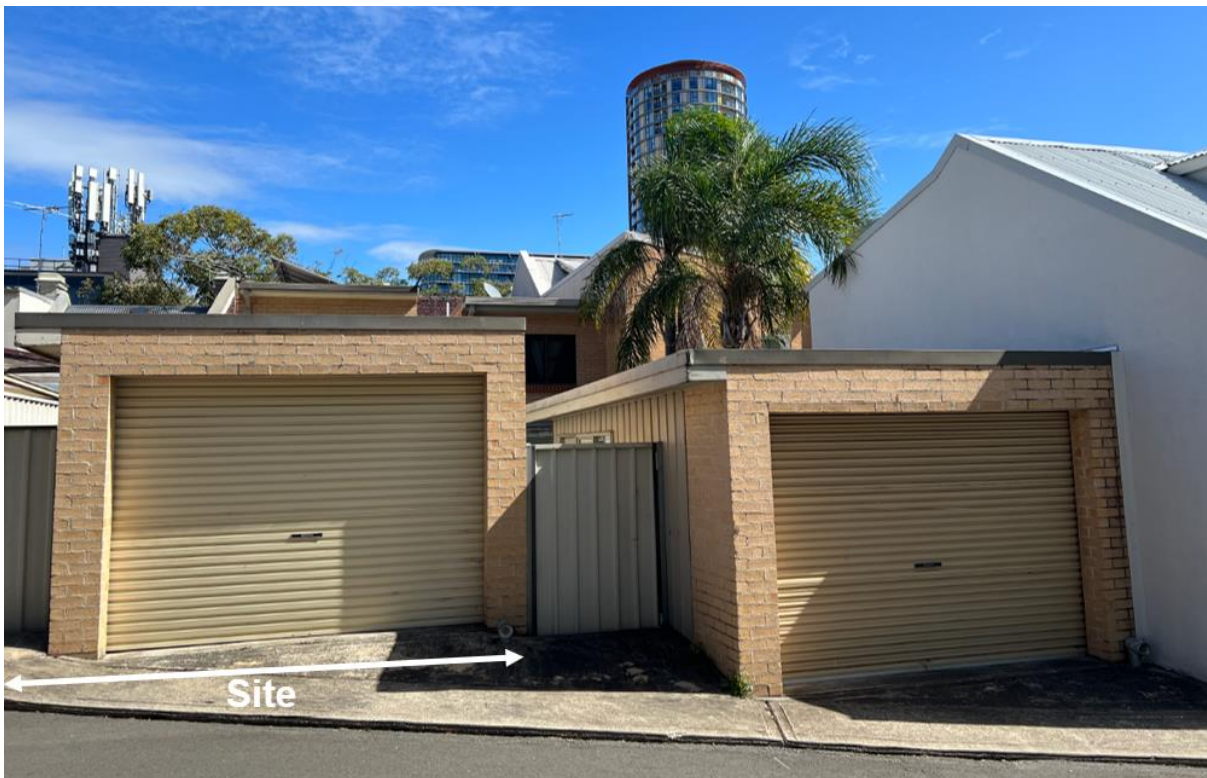
Figure 3: Site viewed from McPherson Lane
